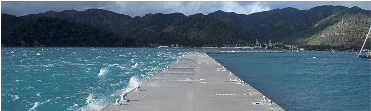
Figure 5: View of floating breakwater attenuating effect.
