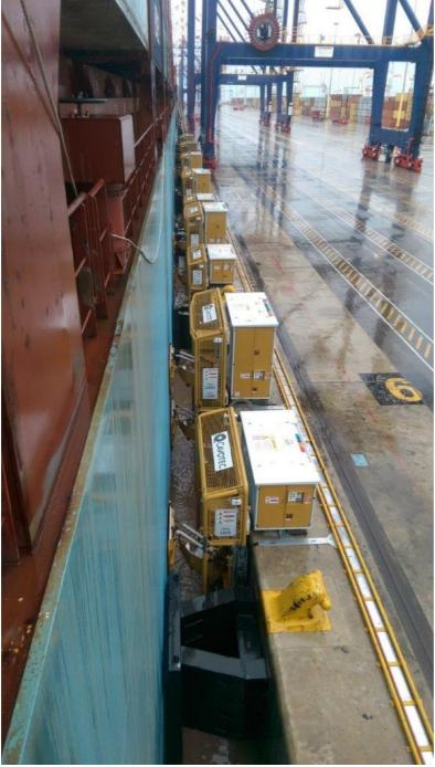
Cavotec MoorMaster™ MM200C<sup>17</sup> system installed in the Port of Ngqura
