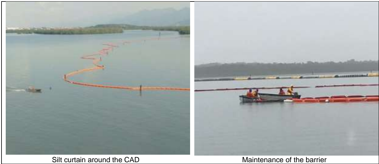
Figure 5: Silt curtain implanted around the entire perimeter of the CAD to control the dispersion of suspended solids.
