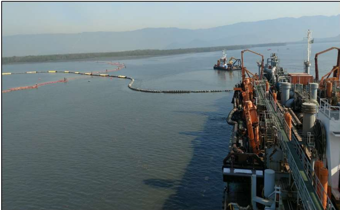
Figure 7: TSHD performing pumping through PEAD piping to fill the CAD.
