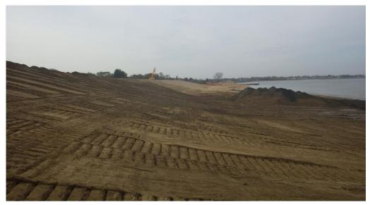
Figure 6 - Construction of beach-fill berm
