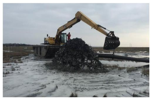
Figure 9 – Pumping Dredged Material onto the Marsh during Fortescue TLP
