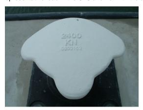
Figure 6. Standard 2400 kN bollard Rotterdam
