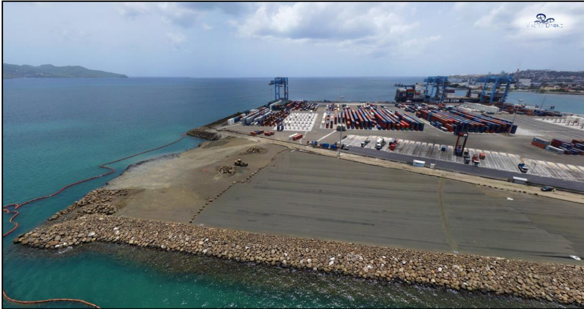
Figure 12: Platform capping and surface dressing layer works (photo: Mad'In Drone (2015))
