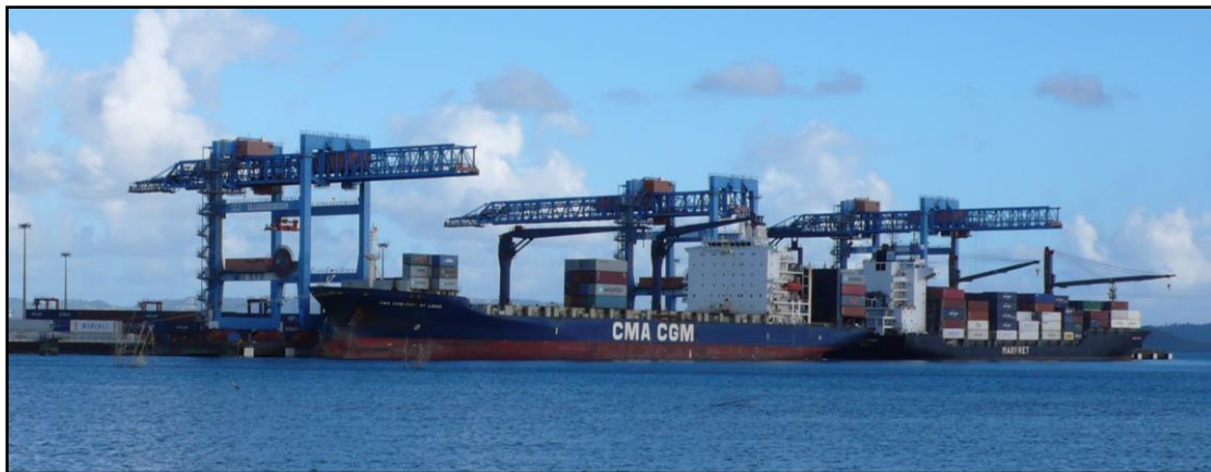
Figure 4: Two CMA-CGM vessels berthed at Pointe-des-Grives (photo: Artelia)
