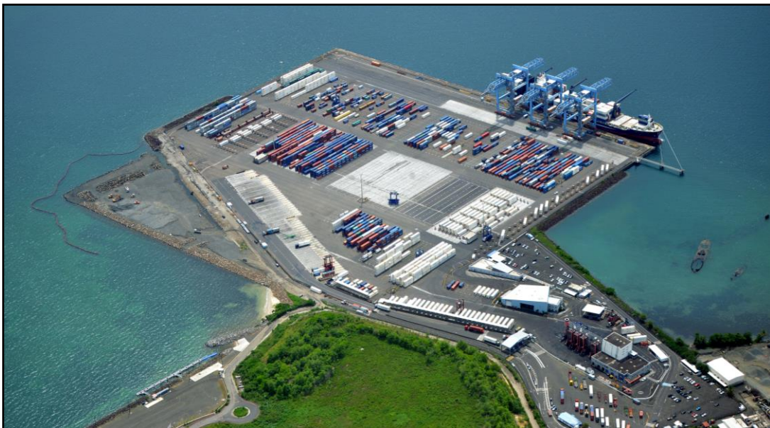
Figure 5: Overall aerial view of terminal during the works (photo: GPMLM)
