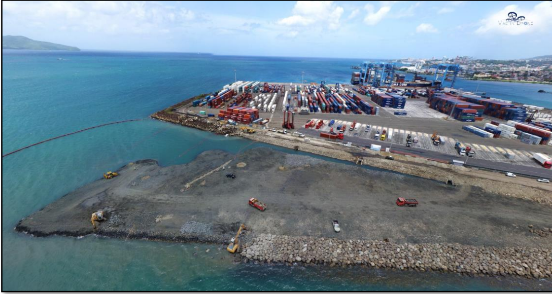
Figure 10: Aerial view of the first work phase (photo: Mad'In Drone (2015))
