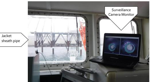
Figure 5: Jacket Induction with the help of surveillance camera
