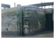
c) Diagonal crack near a corner due to shifting towards the river
