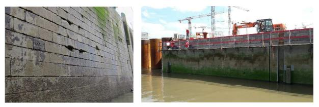
Figure 8: Original bluestone facing (left) and new concrete molded formwork with on top three rows of reused blue stone blocks (right)
