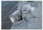
f) Damage to the curbstone as a result of collision with moored ships
