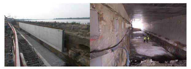
Figure 16: View of the chamber front wall placed on the existing quay wall (left) and view inside the stress relieving chamber (right)
