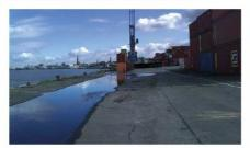
e) Subsidence on the quay due to movements of the quay wall and heavy loads
