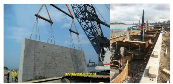
consequently concrete is poured in steps of 1.0 meter. Before each pouring phase previous concrete surfaces and rebar are cleaned. The bollards are integrated in the concrete capping beam.
