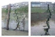
a) Cracks near the juncture between two caisson walls
