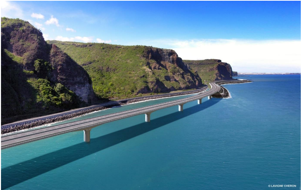
Figure 11: Artist impression of the new highway which will be partly constructed as viaduct and partly as causeway.
