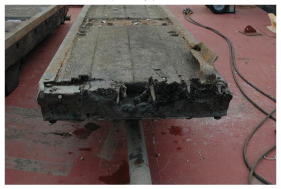
Figure 4: Deteriorated Timber Wicket Gate
