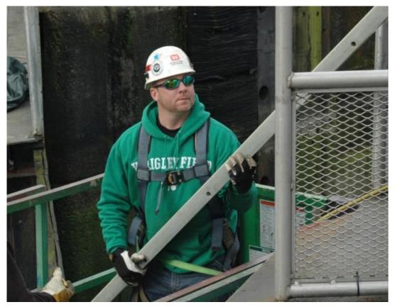
Figure 3: Field Personnel Handling FRP Miter Blocks
