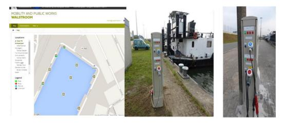
Figure 2. Shore power installations (low voltage) at quay 75 in Port of Antwerp
